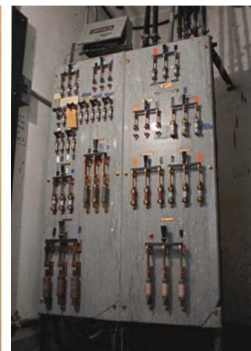
An original fuse box (left) and original electrical switchboard (right).
